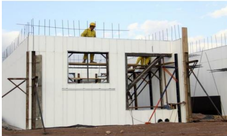
Figure 1: stages of constructing walls based on ICF method (source: mapsa.co.ir)
