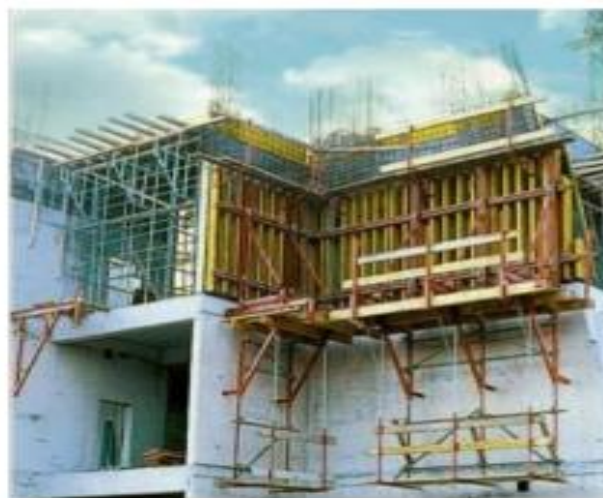
Figure 2: concrete molding
