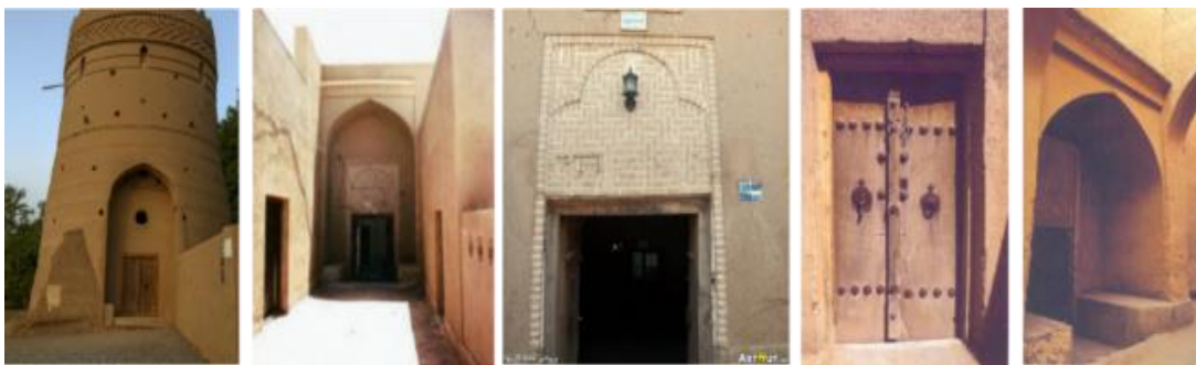
Figure 8: Set back entrances with a distinctive facade from the mud wall to create physical security against climatic factors and psychological security along with social interactions.
