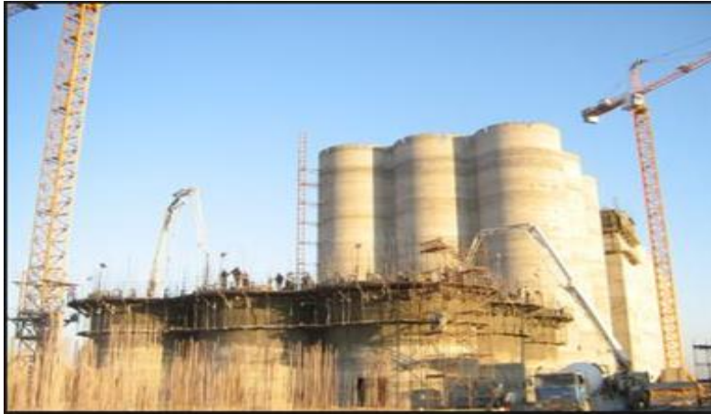
Figure 4: using concrete pump at low height 7
