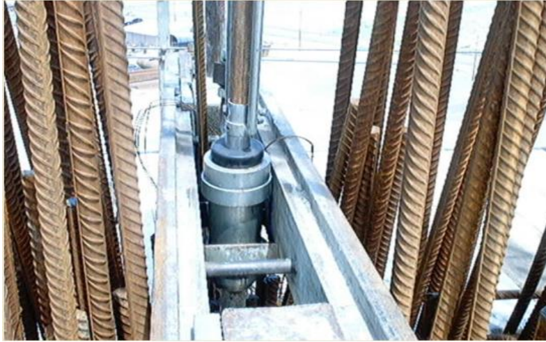
Figure 6: hydraulic power room 11
