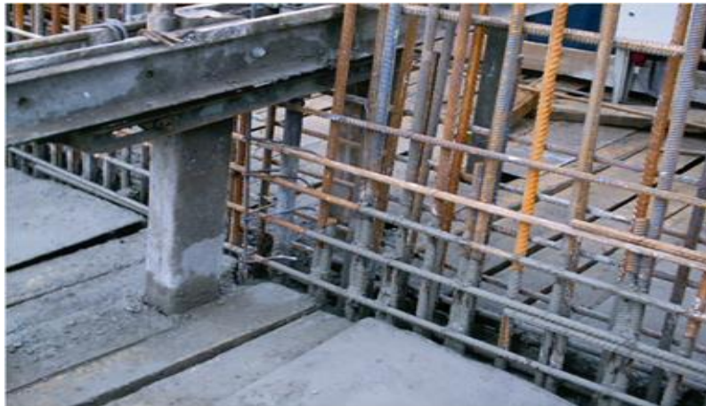
Figure 3: install rebar up to yoke 6
