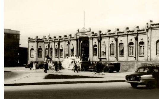
Fig. 4 Shahr bani (Police) Building, Tabriz, present-time Shohada St., 1963 (Source: Jadid al-Islam Personal Archive)
