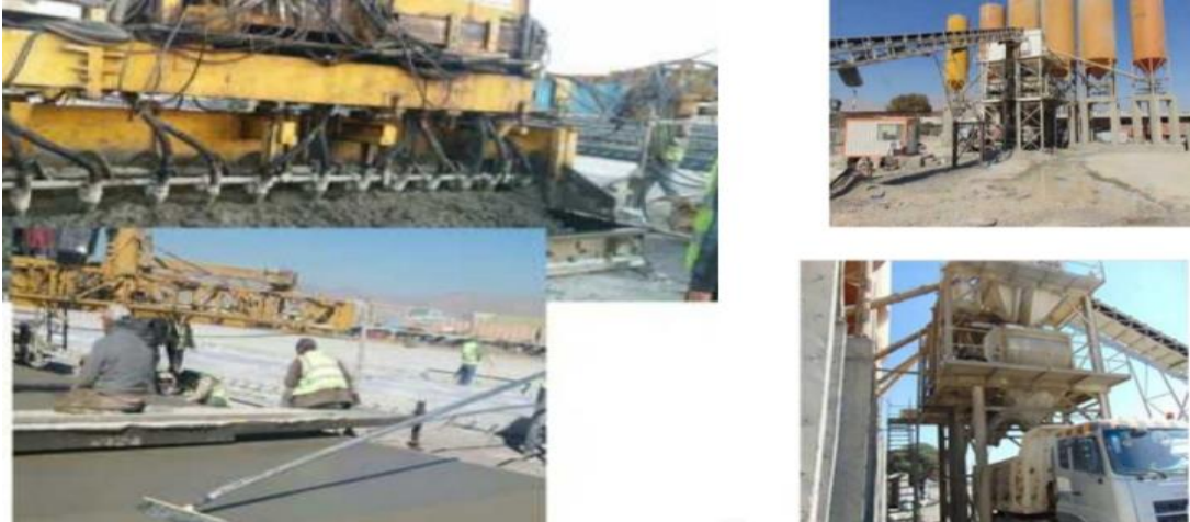
Concrete pavement of Mehrabad airport in Tehran www.imenrah.com 1010-09
